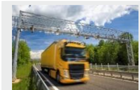
Nationwide truck tolling system (MLFF) in Slovenia
