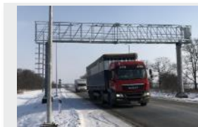
High-speed weigh-in-motion with enforcement in Ukraine
