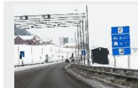
Toll collection systems (MLFF) in Norway
