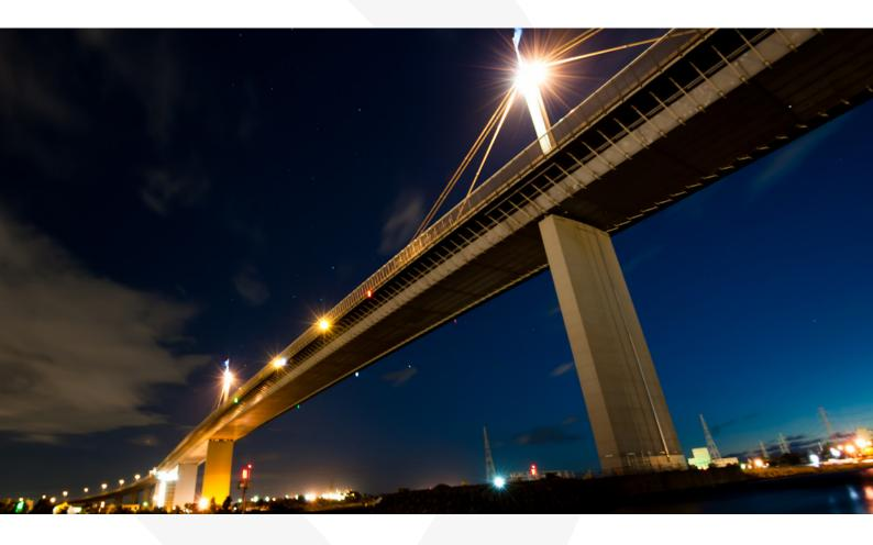
The West Gate Bridge in Melbourne, Australia is a steel box girder cable-stayed bridge and was originally designed to carry 40,000 vehicles per day with a maximum load of 25 tonnes per vehicle. Today, traffic volumes are now 160,000 vehicles per day with some B-double trucks weighing up to 68 tonnes each.
